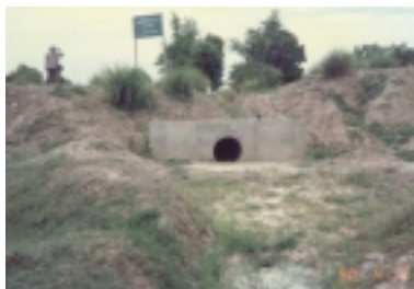
Figure 1: Concrete pipe through embankment
