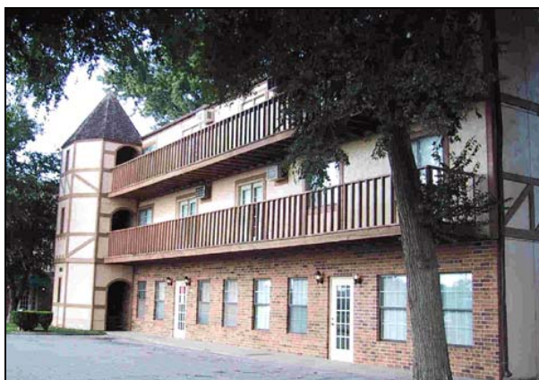
Alexis Park Inn and Suites adjacent to the Iowa City Airport
