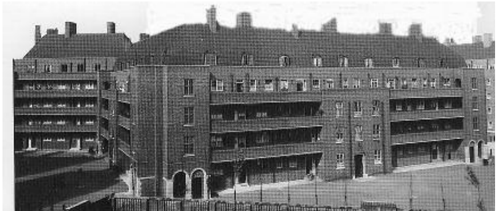
LCC Council Flats (Slum clearance)
