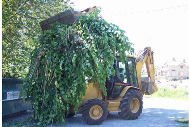
Heavy equipment at work
