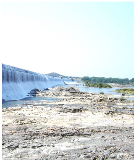
Dukwan dam site
