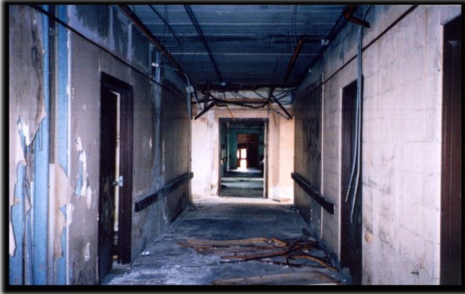
The Main Hallway. The railings on the walls were one of the last things to be added to the structure.
