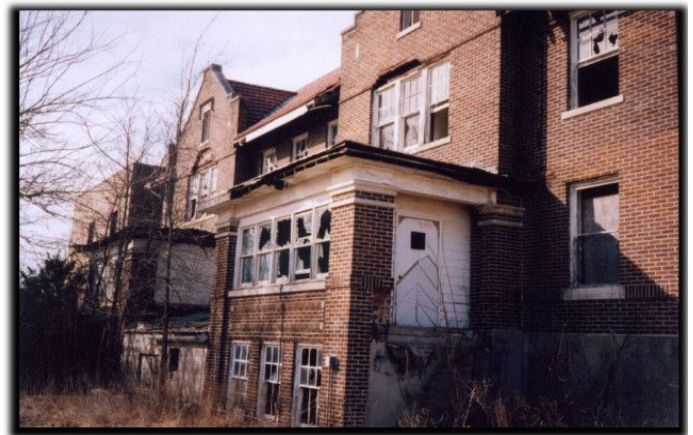
Top: Fall has revealed more of the front structure.
