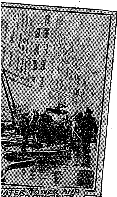
Water Tower and Ladder Opposite Building in Washington Place.
