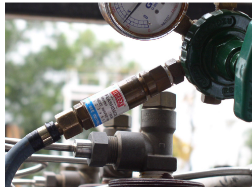
Figure 4 Flashback arrestor fitted at the outlet of a pressure regulator
