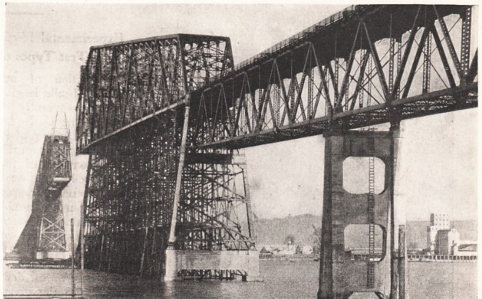
FIG. 3—LONGVIEW BRIDGE PROVIDES 195-FT. VERTICAL CLEARANCE UNDER MAIN SPAN
