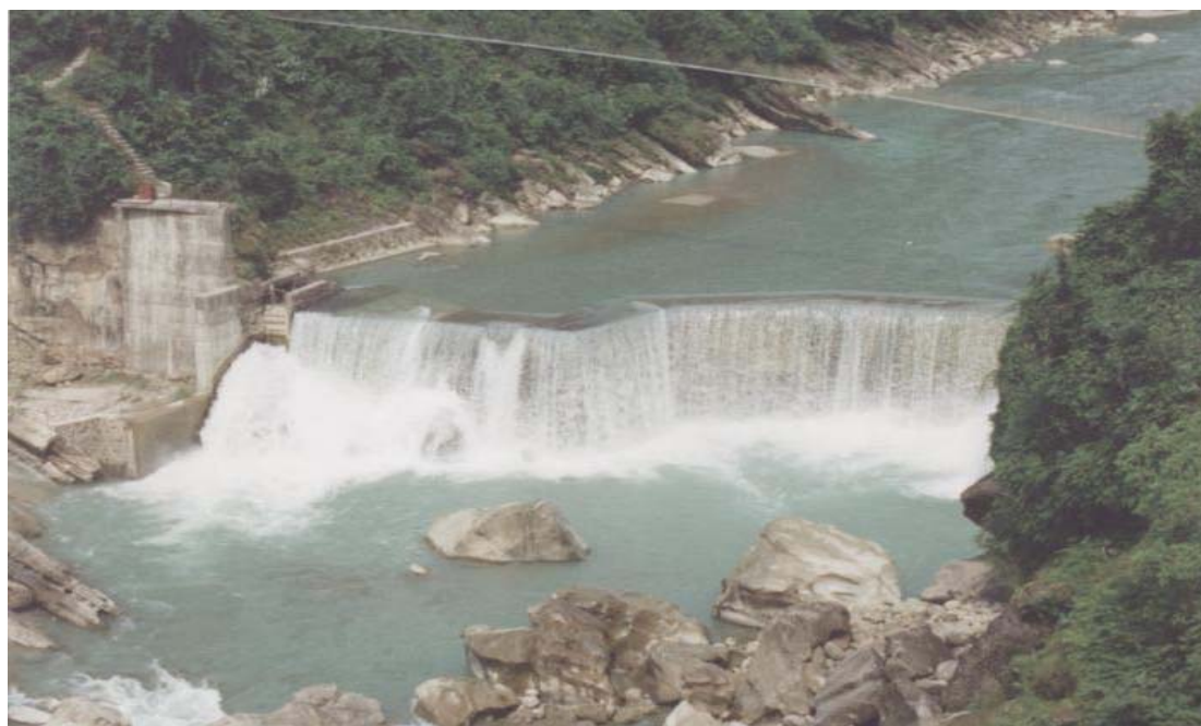
Fig 1. Eight meter high Tinau River dam without impoundment (photo taken in October 2002).
