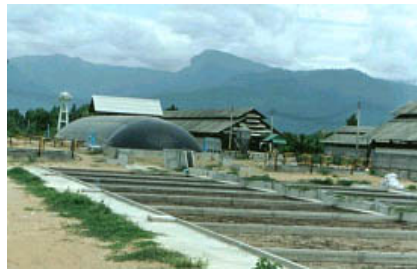
Fig 7: C.P. Chomthong Farm's biogas plant [2]
