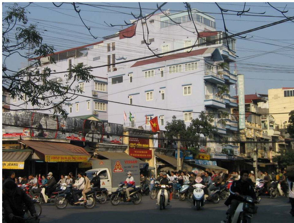
Figure 1: This light-blue multi-story building is made of two conjoined buildings. The shorter one in the foreground is the Pacific Star Hotel. We stayed on the 3 rd floor in the taller one in the background, which is the Pacific Hotel.
