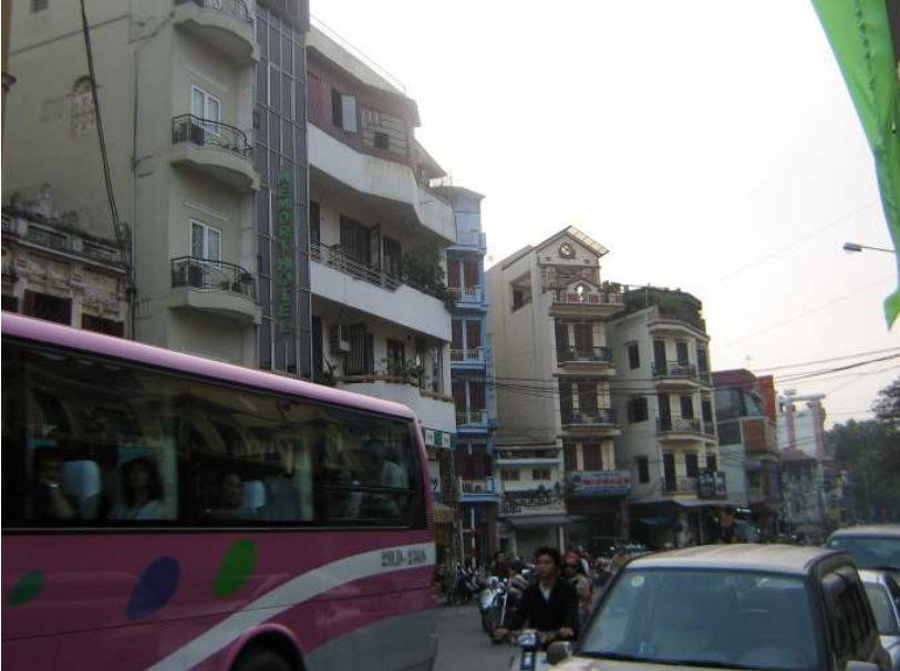
Figure 4: Land for buildings seem to be a premium in Vietnam, both in the countryside and in the cities, as most private lots are quite small in area. As a result, many buildings are taller than they are wider, as seen in this shot of a typical street in Hanoi.
