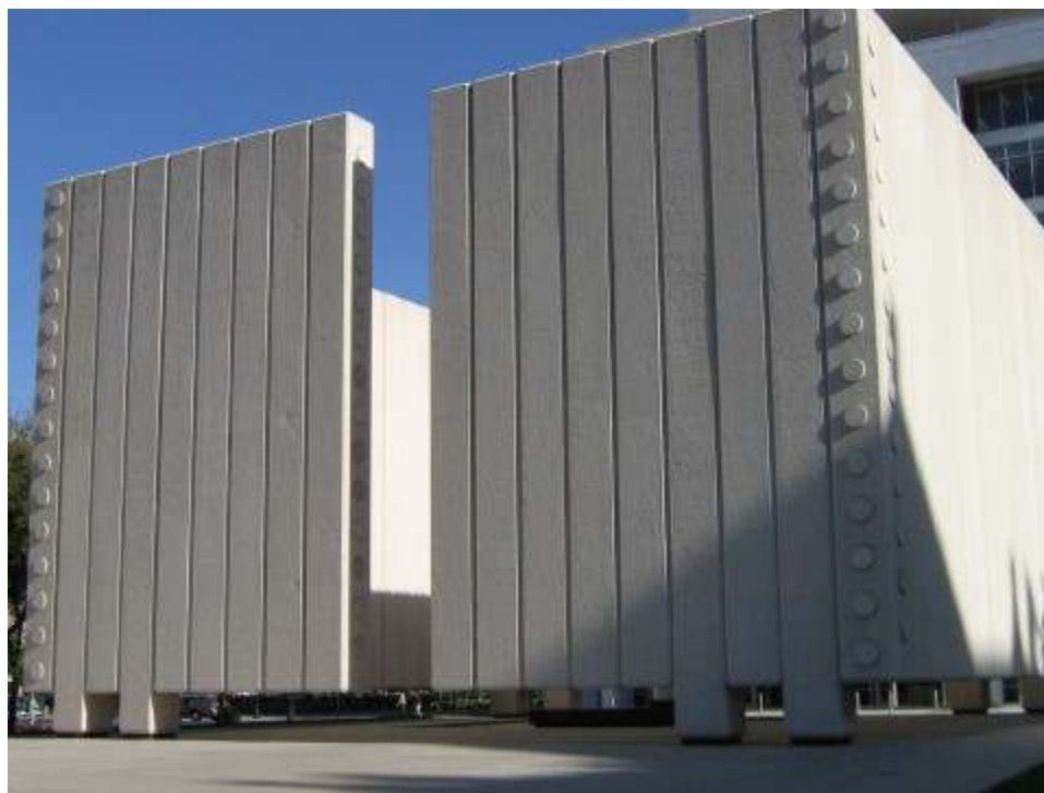
Figure 6: It's a space for contemplation, neither open nor closed. The 50 foot square enclosure with 30 foot high concrete walls would be oppressive, if not open in the center of two opposite walls and along almost the entire base
