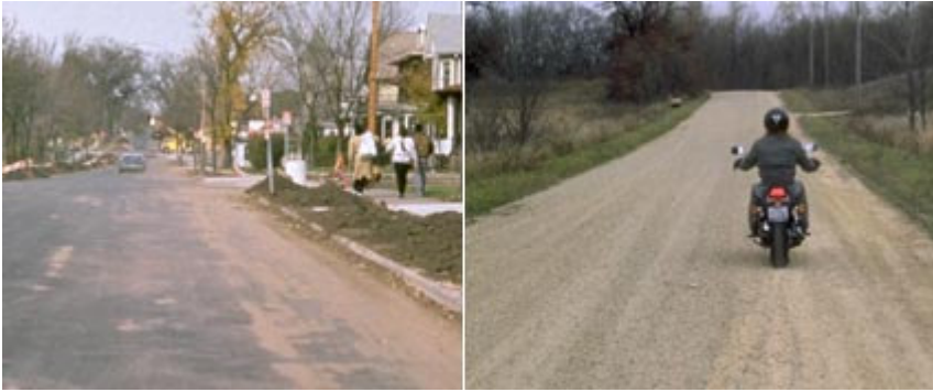
- Edges of roadway.
