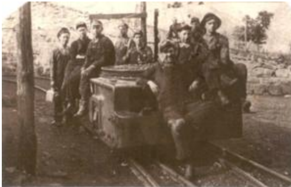
Photo 18: Miners coming up from Mine Shaft on Mine Motor Car (11)
