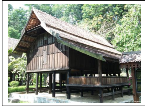
Figure 2 'Rumah ibu' with higher space floor and headroom than other areas (Source: http://teganukita.my/rumah-tradisional-terengganu-dipindah-ke-muzium-warisan-upm )
