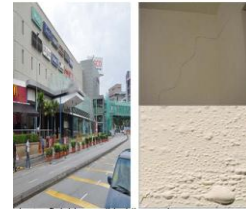
plaster finishing wall building at damansara utama
