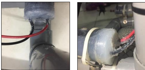
Figure 3.5: Waterproofing the motors
