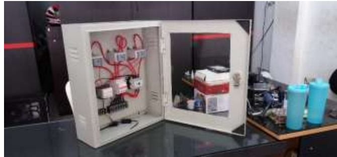
Figure 3.4. Protection device that is ready to be installed
