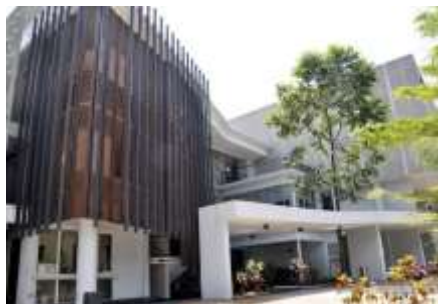
Figure 6: West-facing “double-skin” facade minimises heat gain into the building.
