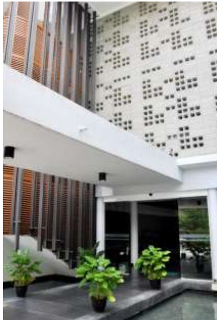
Figure 7 Pot-holed block walls provide natural ventilation throughout the building while water features and greenery complement the entrance
