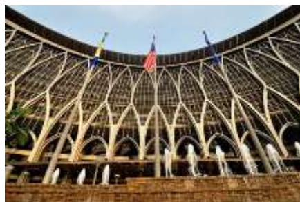
Figure 8: Sun shading devices integrated with traditional motif as architectural design expression for the Malaysian Ministry of Finance building in Putrajaya, Malaysia
