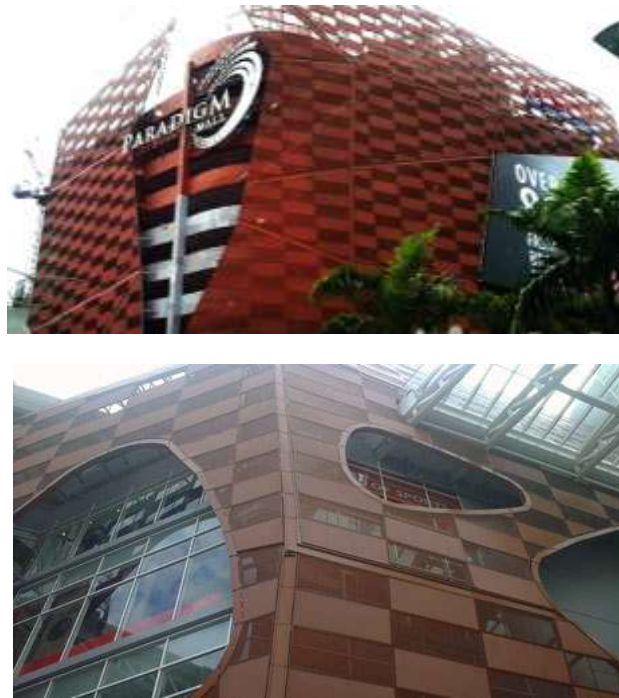
Figure 9 (a) and (b) : Complex Façade system in Paradigm Mall, covering and filtering the direct sunpath to the carpark and part of the offices.
