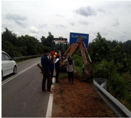
Fig 3.3 Site in clearing process
