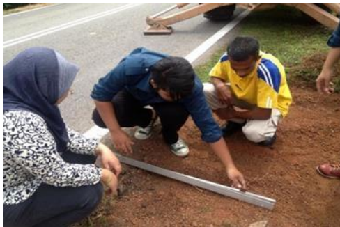
Fig 3.4 Product testing on site
