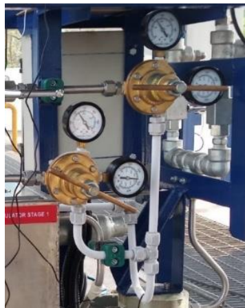
Figure 17. Joule Thomson Effect phenomenon that occurs when gas flows from the Stage 1 regulator when the gas is lowered from 250 BAR to 15 BAR with flow-rate 102 Nm 3 / h.
