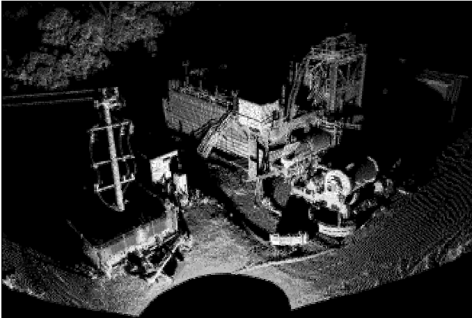
Figure 4. Perspective view of an I-SiTE scan from a mine's surface infrastructure.
