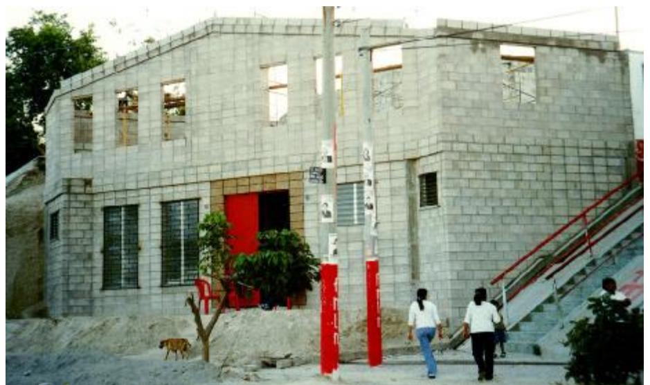
Santísima Trinidad Church and Youth Centre in final stage of construction
