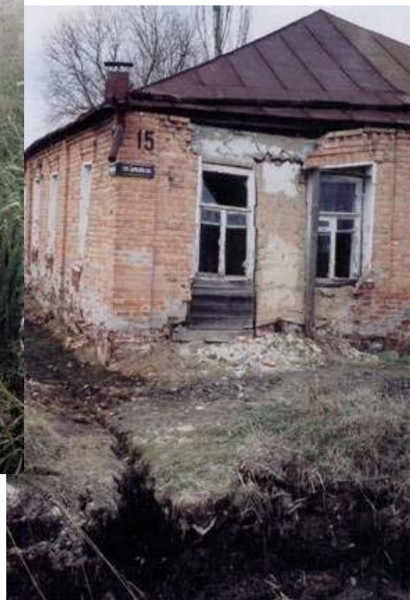
A house that has been damaged by the slow flooding
