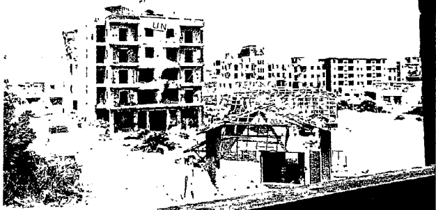
A UN observation post in the city of Suez, destroyed during the October War
