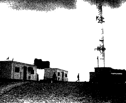
Sector control center in the Fiji sector
